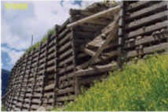
Based on this information, a temporary Mechanically Stabilized Earth (MSE) “deep patch” system was designed to mitigate the settled lane of U.S. 40 for approximately one year. This required closing all but one lane of U.S. 40 in order to excavate the settled section of highway and remove and replace and crib wall with a modular block MSE wall. The work was done between Sunday and Thursday to reduce adverse impacts to the heavy summer tourist traffic during the weekend.
