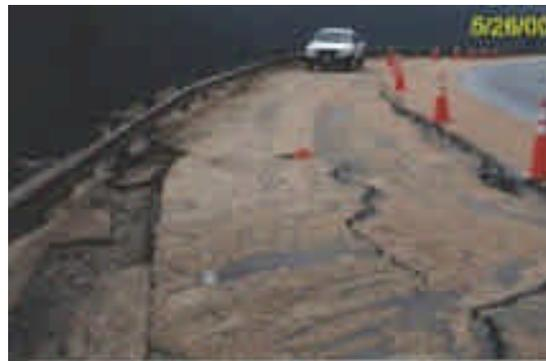
Department of Transportation (CDOT) to close one lane of the highway indefinitely. The settlement was directly caused by the overturning failure of a section of the existing foundation retaining wall. The wall is
