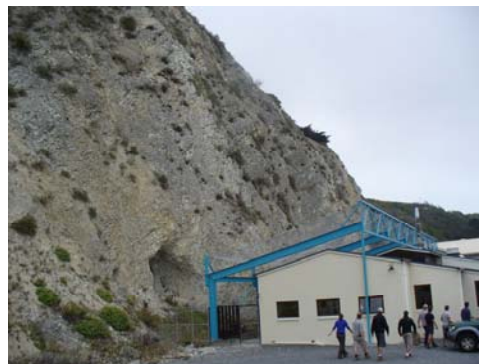
Rockfall protection system over faculty housing at Kaikoura field station
