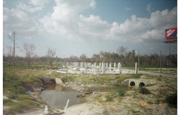
The 9<sup>th</sup> Ward in New Orleans. Destruction here was mainly due to failure of sheet-pile walls along the Industrial and other canals. This resulted in widespread flooding which affected large parts of the city. Due to its proximity to the breach in the Industrial canal, the destruction in the 9<sup>th</sup> Ward was compounded by rapidly moving water. In other places, the destruction was confined to water damage.
