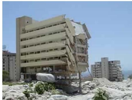
\*Apartment in Caraballeda extensively damaged by passage of debris-flow front at least 3.5 m in height, leaving boulders (> 1m) on second floor of structure.\* Source: <http://pubs.usgs.gov/of/2001/ofr-01-0144/Venezuela/image033.jpg>, accessed May 18, 2006.
